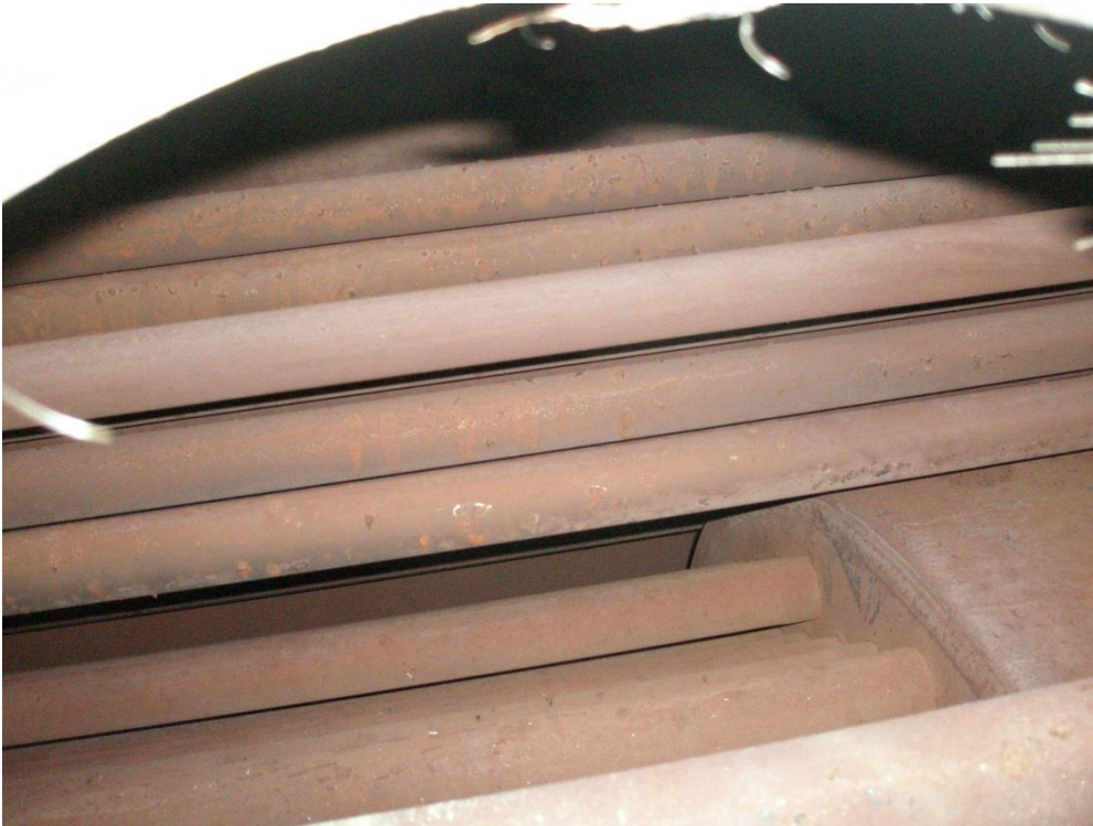
Boiler 2 Second and third pass tubes and rear smoke box from top manway. June 2013
