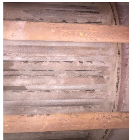
Boiler 2. Second and some third pass tubes and rear smoke box from top manway. June 2017
