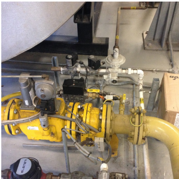
Typical Boiler installation with its gas supply.
