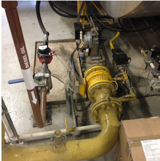
Above: Multiple fuels - Diesel and Gas valves for an industrial boiler.
