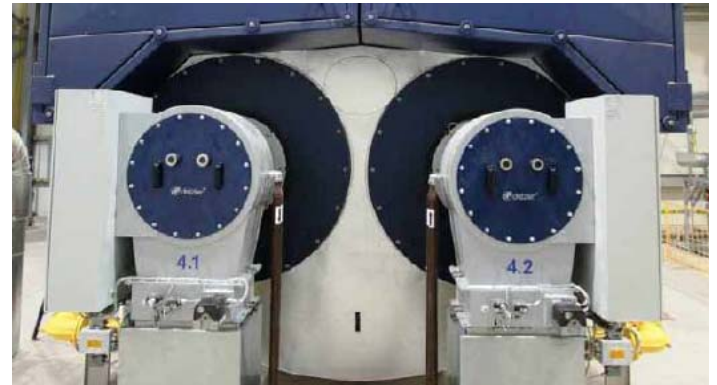
Boiler 4 2 x marathon® MC 10003.5 ARZsuper Combustion capacity 17 MW with Loos double flame tube boiler UT-HZ 32500x18
