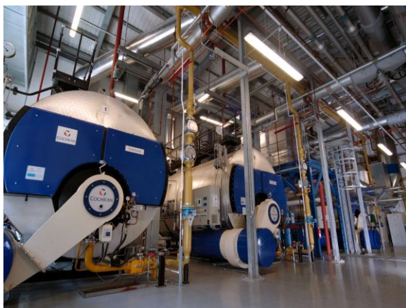
Inside the hospitals energy centre two of the three Cochran boilers and CHP engine.
