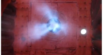
When considering a new fuel in a boiler, including  $H_2$ , a boiler impact study can highlight any impact on boiler performance. The combustion characteristics of  $H_2$  can lead to changes in where and how radiative and convective heat transfer occurs within the boiler, which may adversely impact steam generation rate and steam temperatures.
