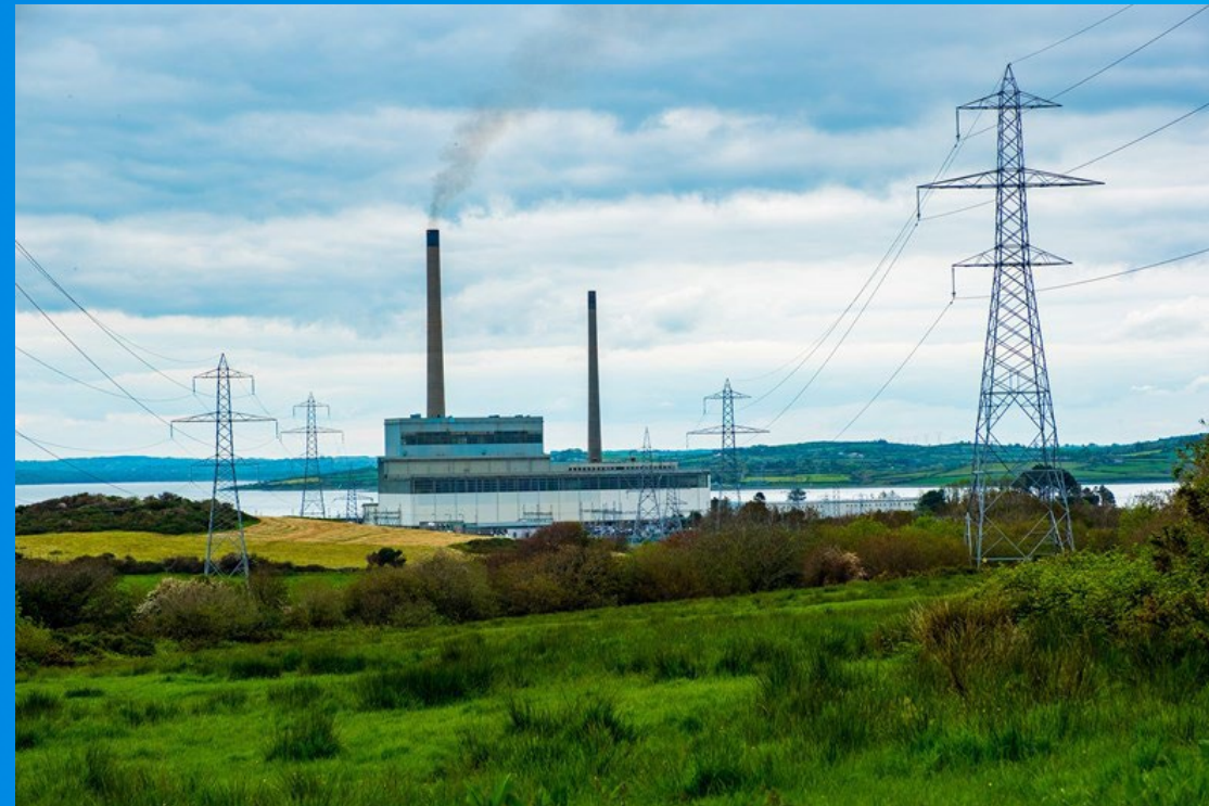
Platin Power Station [4]
